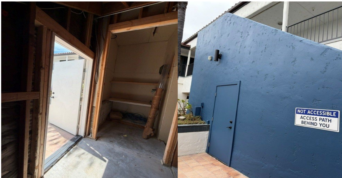
STORAGE AREA ACCESS
