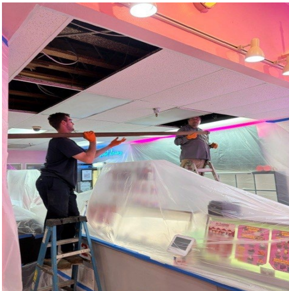
CAST IRON PIPING WAS REPLACED
