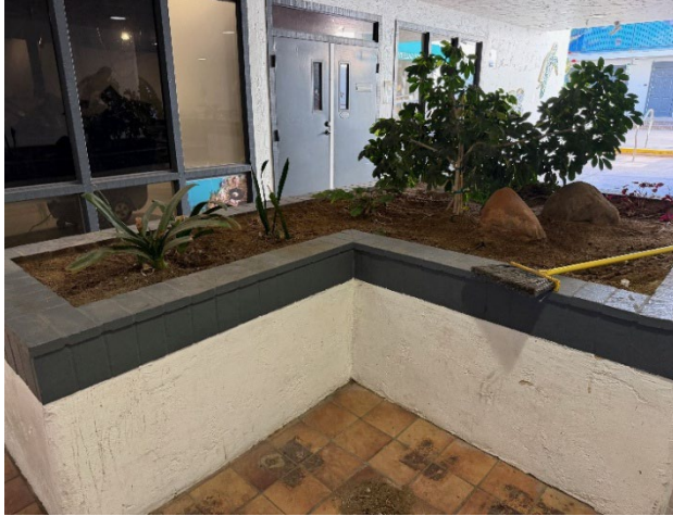
Planter Improvement in Process
