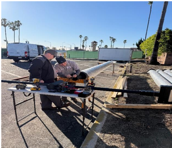
Light pole head assembly
