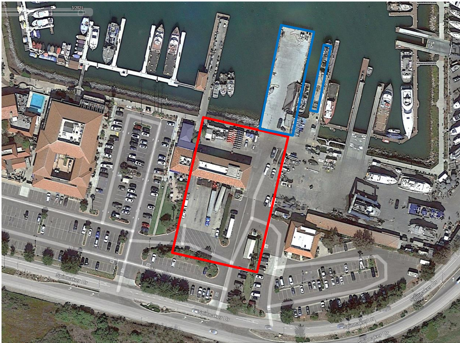
Current Ventura Port District's Commercial Squid Offloading Pumps (Blue) and Sorting Facility (Red)
