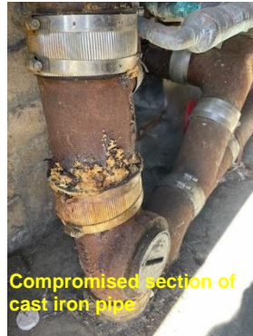
Replaced plumbing pipe with ABS
