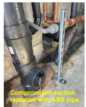
Compromised section of cast iron pipe
