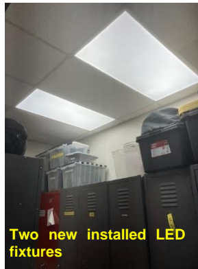
Installation of new LED fixture
