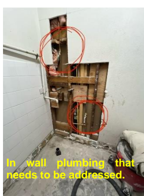
Demo of the removed sink, plumbing and floor tile
