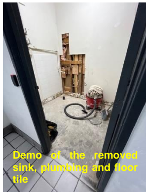
In wall plumbing that needs to be addressed.
