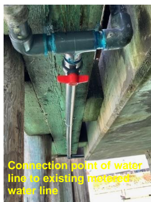
New installed water line mounted under fish pier.
