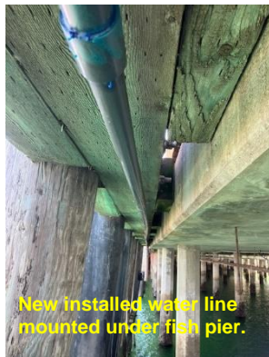
New installed water line mounted under fish pier.
