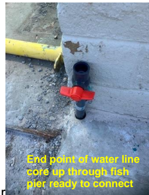
New installed water line mounted under fish pier.
