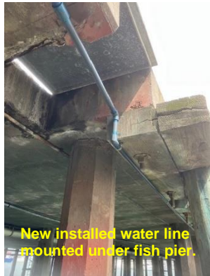
New installed water line mounted under fish pier.
