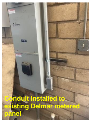
New conduit run from Delmar panel to exterior wall
