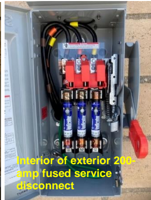
480V 3-phase service disconnect ready for ice machine install.
