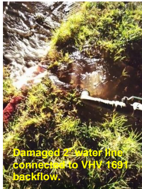
Crew removing damage backflow and initiated repair.
