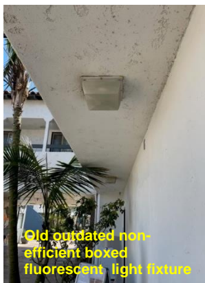
Old outdated non-efficient boxed fluorescent light fixtures
