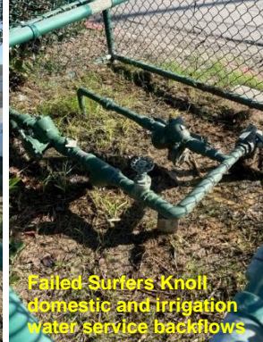
Replaced Surfers Knoll domestic and irrigation water service backflows
