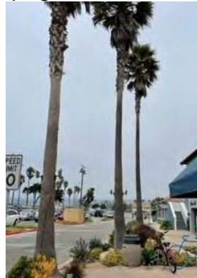
Installation of new up-lights
