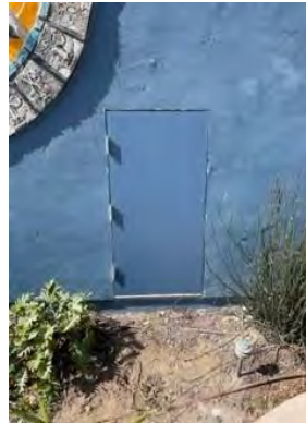
Custom door installed on exterior
