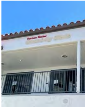
2 nd floor signage removal
