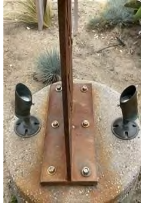
Installation in progress at VHV promenade
