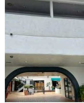
1 st floor signage removed and repaired
