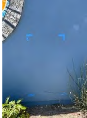
Marked area for exterior door
