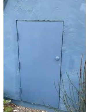
Progression of exterior Install
