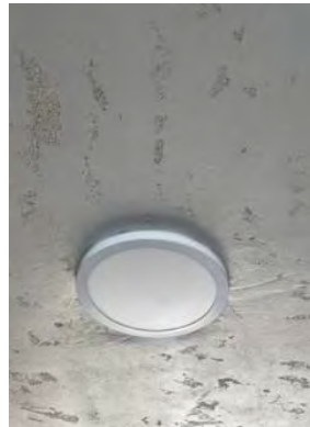
Replaced newer efficient LED fixture
