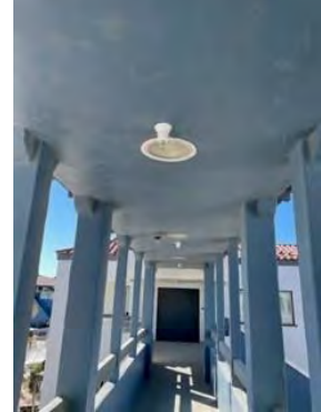
Replaced escutcheons and skirts on hallway
