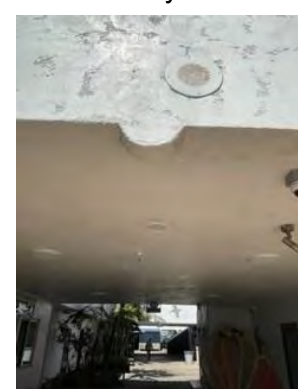
Replaced fixtures at south courtyard eve
