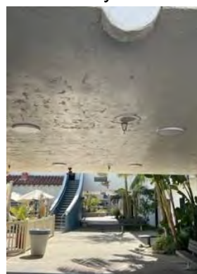
Replaced fixtures at north courtyard eve
