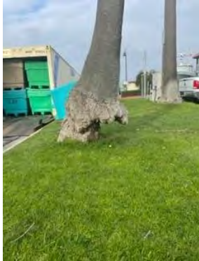
Base of unsafe palm at 1431
