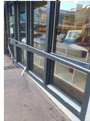
Repair in progress
