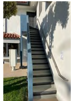
Staircase to be cleaned
