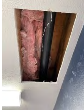
Pipe replaced w/ABS
