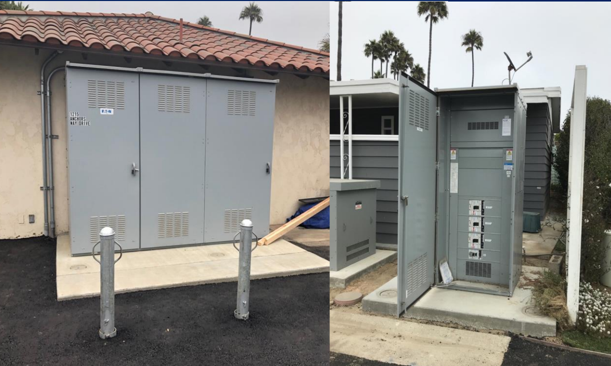
New Main 1,600 Amp & 600 Amp Switchboards
