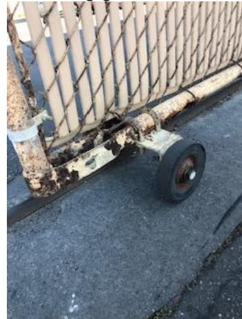
Old rolling gate failure
