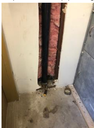
Replaced ABS pipe to ground
