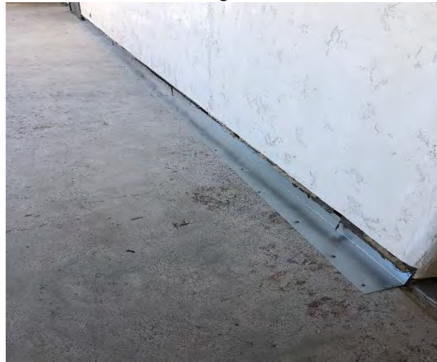
New flashing
