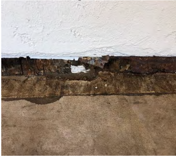
Failed flashing
