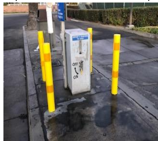
Repainted bollards with reflective tape
