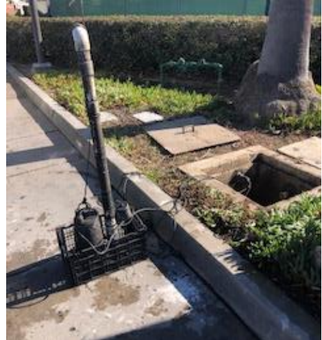
Defective sump pump
